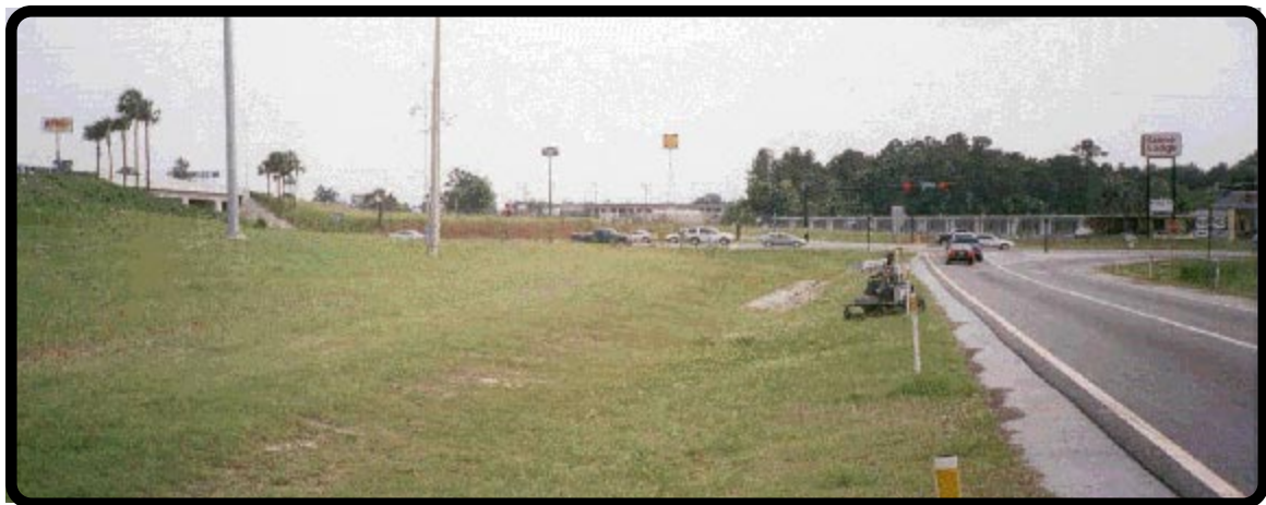
The NW Quadrant of the US 90 Interchange as it exists today
