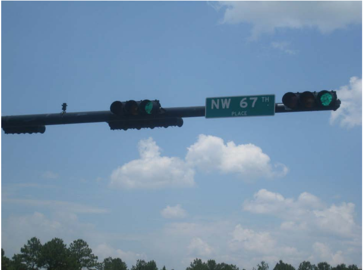
Figure 9 - Mast Arm with Horizontal Signal Heads
