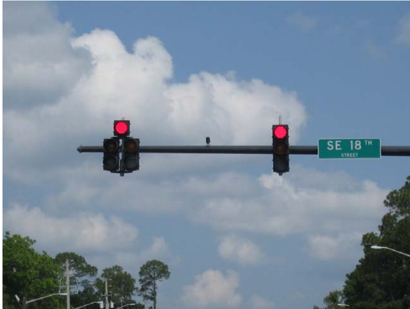
Figure 10 - Mast Arm with Vertical Signal Heads
