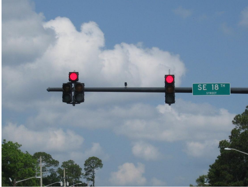
Figure 10 - Mast Arm with Vertical Signal Heads
