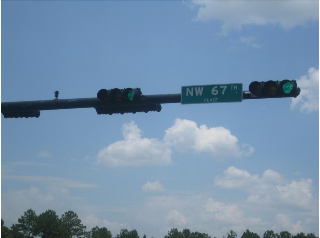
Figure 9 - Mast Arm with Horizontal Signal Heads
