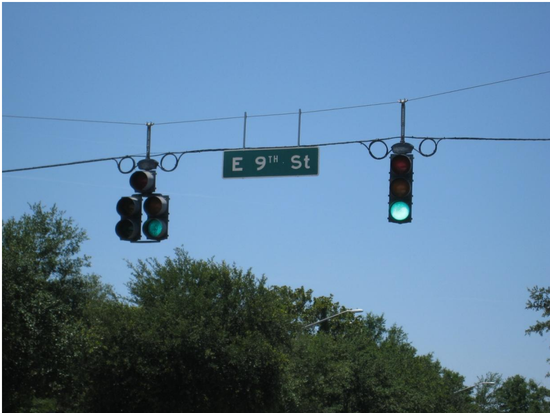
Figure 8 - Strain Pole Traffic Signal
