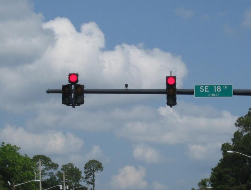
Figure 9- Mast Arm with Vertical Signal Heads
