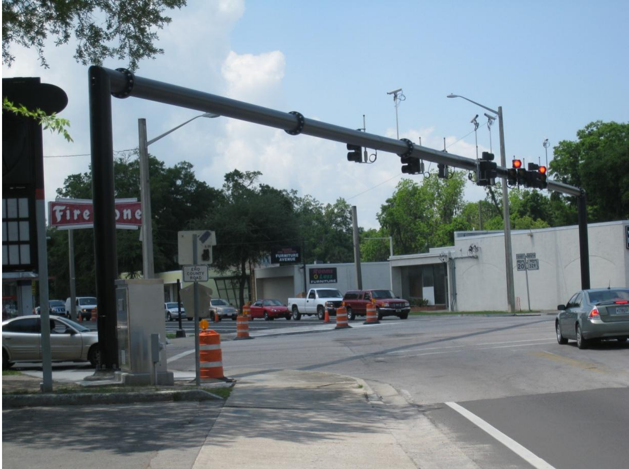
Figure 11- Monotube Mast Arm
