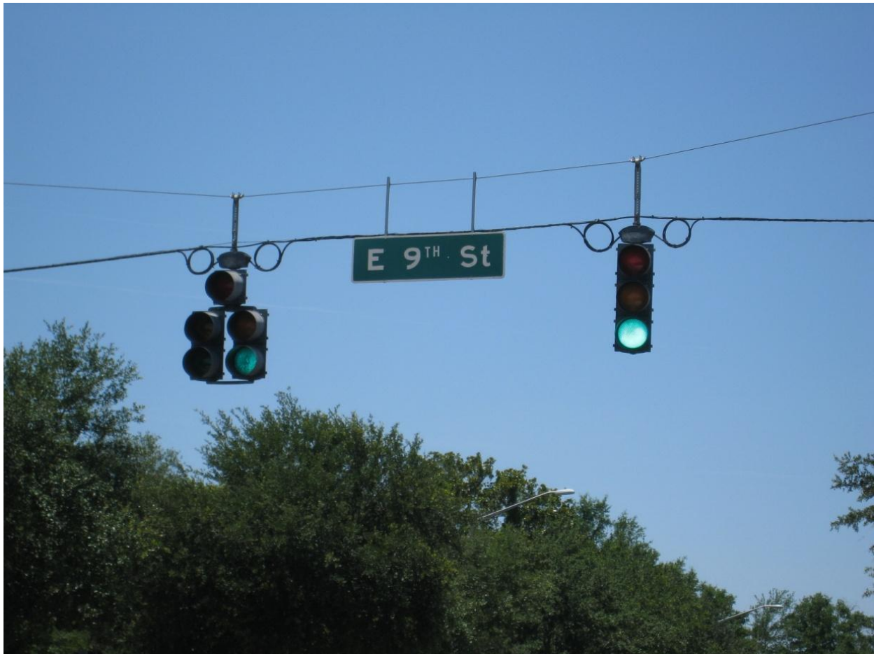
Figure 7- Strain Pole Traffic Signal
